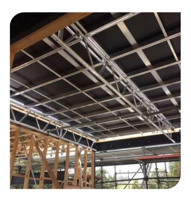
Rated to carry a 225kg Load Limit, Turbo Scaffolding Void Protection ensures that a person cannot fall from above the void area, as well as into the void area. This stair void system allows the area under the void to remain open and clear of scaffolding and comes with a secure ladder that is locked into place. This is the only 100% correct stair void method of filling the void area and required by Industry safety standards.
